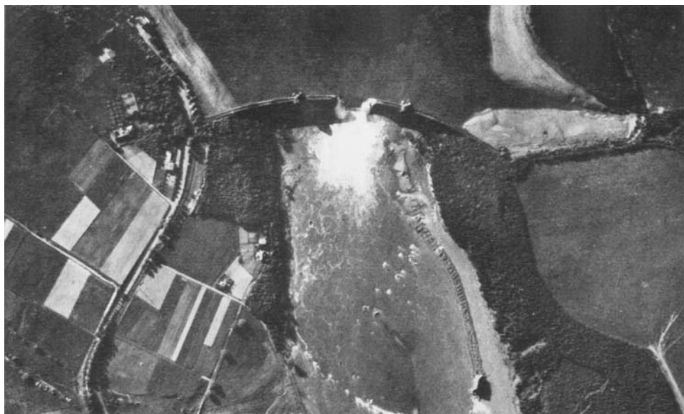
Fig. 17. Damage Done to Moehne Dam by Bomb Attack (Crown copyright reserved.)
